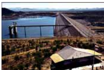
Embankment Dam. Credit: Bureau of Reclamation.
