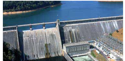
Norris Dam: TVA's first hydro dam. Credit: TVA.
