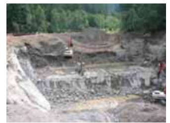
Marmot Dam during demolition
