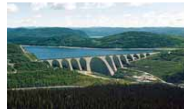
Buttress dam in Canada
