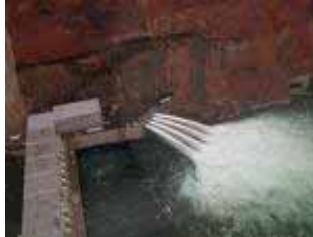
High flow test. Credit: U.S. Bureau of Reclamation.
