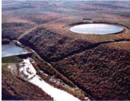
Pumped storage facility in Warren, PA. Credit: FirstEnergy Corp.
