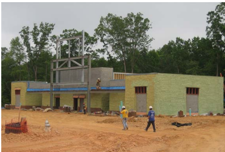
FIGURE 4. Air Barrier on Field House.
