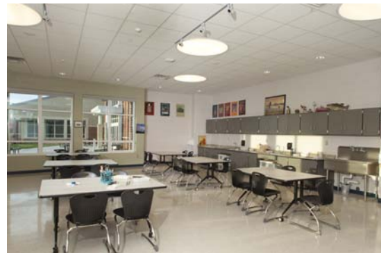
FIGURE 17. Classroom Resilient Floor.
