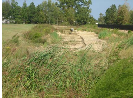
FIGURE 3. Extended Detention Basin.
